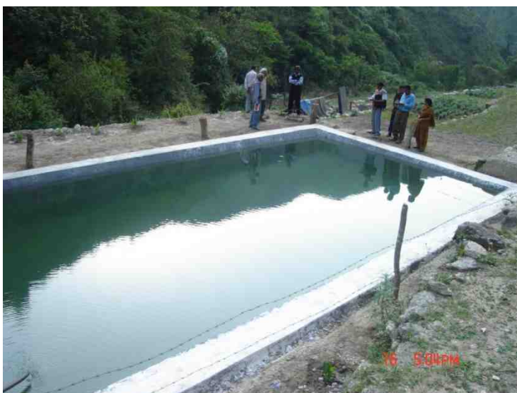
Farm ponds for harvesting runoff and recycling during midterm droughts in Adilabad, Andhra Pradesh and a village pond in Uttaranchal
